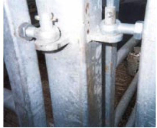
Figure 4: Hinge pintles may need to be moved to allow gates to open fully
